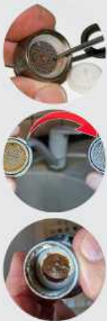
How to remove aerator on the faucet for cleaning
